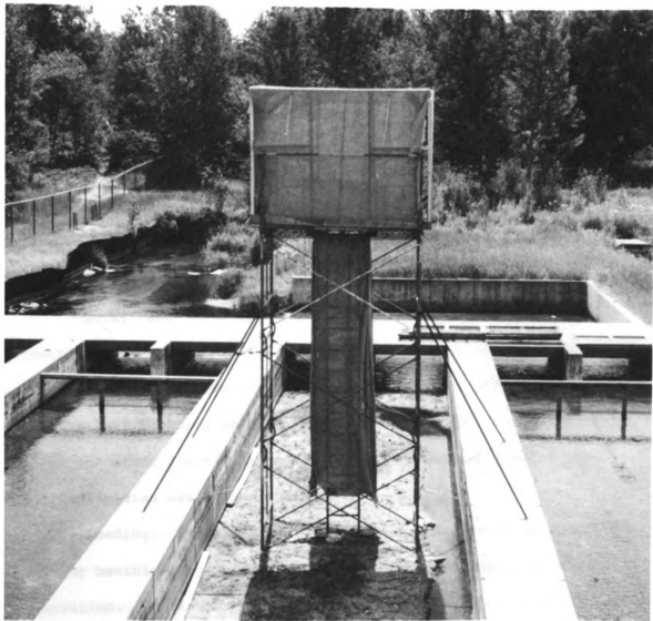
Figure 9. - Side view of the downstream observation blind showing the enclosed ladder and high channel walls. A window faces the channel on both sides of the blind.
