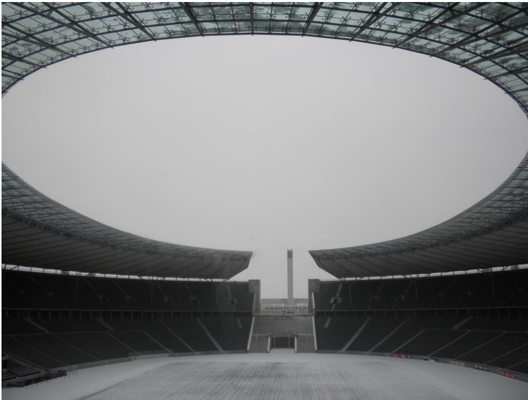
Figure 5.1. The new roof, designed by Gerkan, Marg and Partner in 2004, is open at one end in order not to obstruct the view of the Glockenturm, thereby preserving the stadium's historical design. Photograph by the author.
