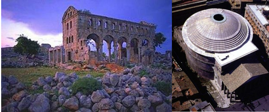
(a) lime-based concrete building in Middle-East (b) Pantheon in Rome made with volcanic ash/lime-based concrete
