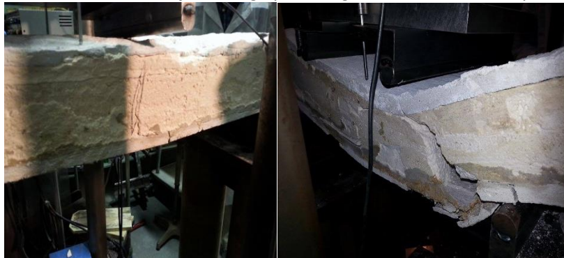
(a) Initial cracking of tension skin
