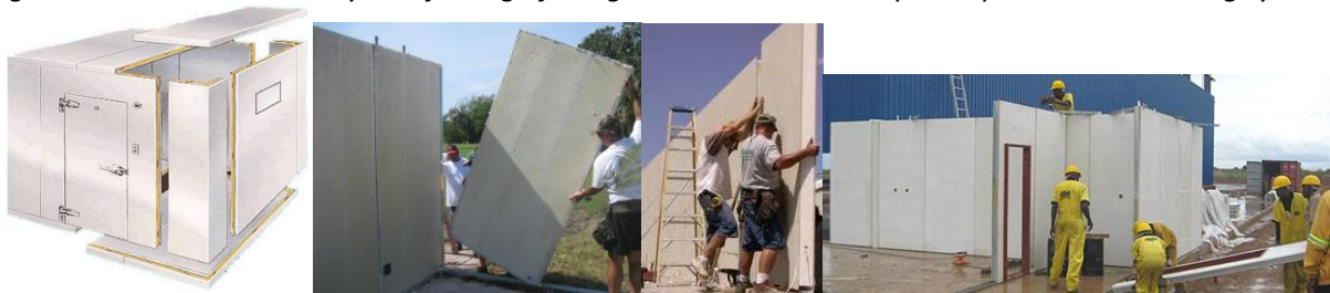
(a) Manual assembly of sandwich composite panels into a building system
