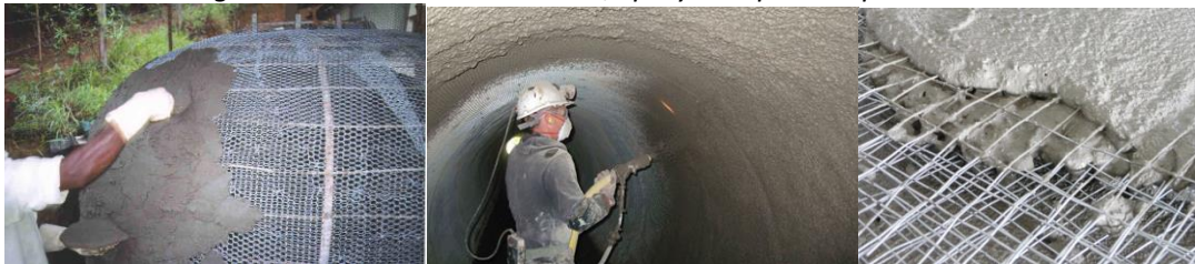
Figure 3.2 Ferrocement trowel, spray and precast production.
