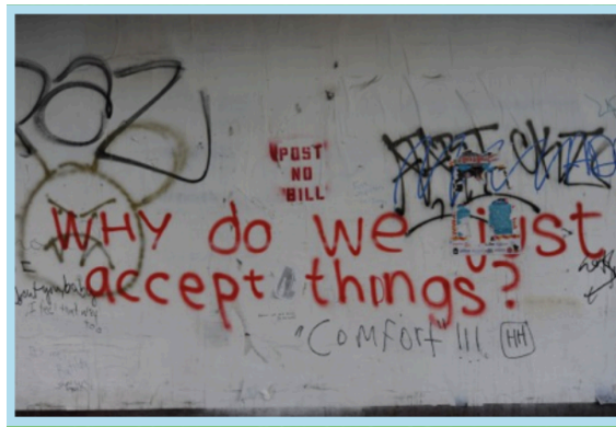
Figure 17: Kilgore Community Bridge Tagging
