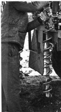
Figure 5. Drilling first auger section into the ground.
