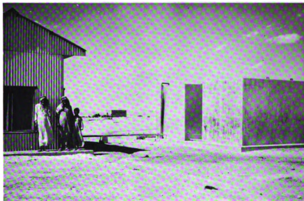
Fig. 1. -- An idle government-drilled well in the northern section of the Western Desert. At the time of the picture (Sept. 20, 1963) the engine in the pump-house to the left was broken, and ten of eleven nearby dwellings were vacant because of lack of water.
