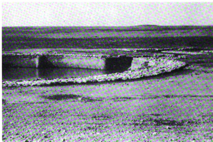
Fig. 2. -- Birkat Hamad, one of the masonry-lined tanks along the Darb Zubaida. It is about 100 feet in diameter and 30 feet deep. Notice flatness of the desert (Ralph M. Parsons Co.).
