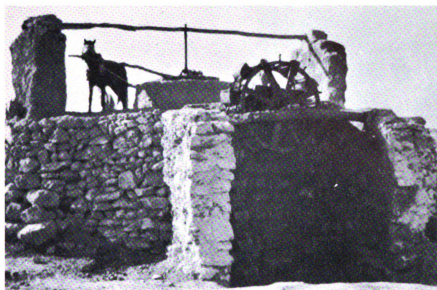
Fig. 1. -- Irrigation na'ur at Dagani in the southern part of the Jezira. Water raised from just below the surface is carried by canal to the village garden plots (Ralph M. Parsons Co.).
