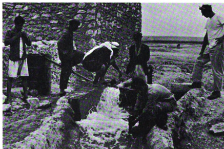
Fig. 2. -- Bir Slubi, a privately owned hand-dug well, in the southern Jezira. The yield of 200 gallons per minute of water having 7,100 parts per million soluble salts is used for irrigation of wheat. (Ralph M. Parsons Co.).
