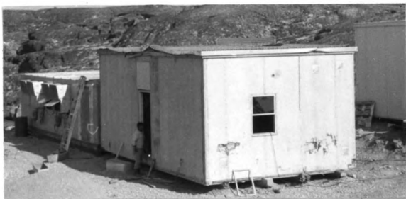
Figure 23.--Construction of the Fish Processing Plant in August of 1971.
