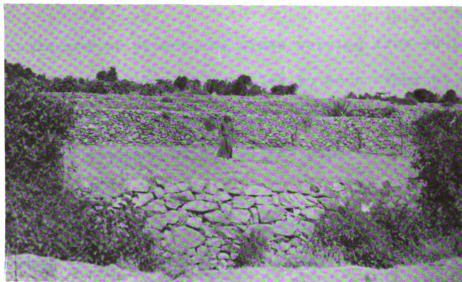
Plate 10a Irrigable terraces on moderate and steep slopes in the Jedaen Mountain, NW of Garen Ben Sahir. The walls are semi-vertical and they usually consist of two rows of boulders with filling of gravels and earth in between. The wall face is smooth and consists of semi-symmetrical materials.
