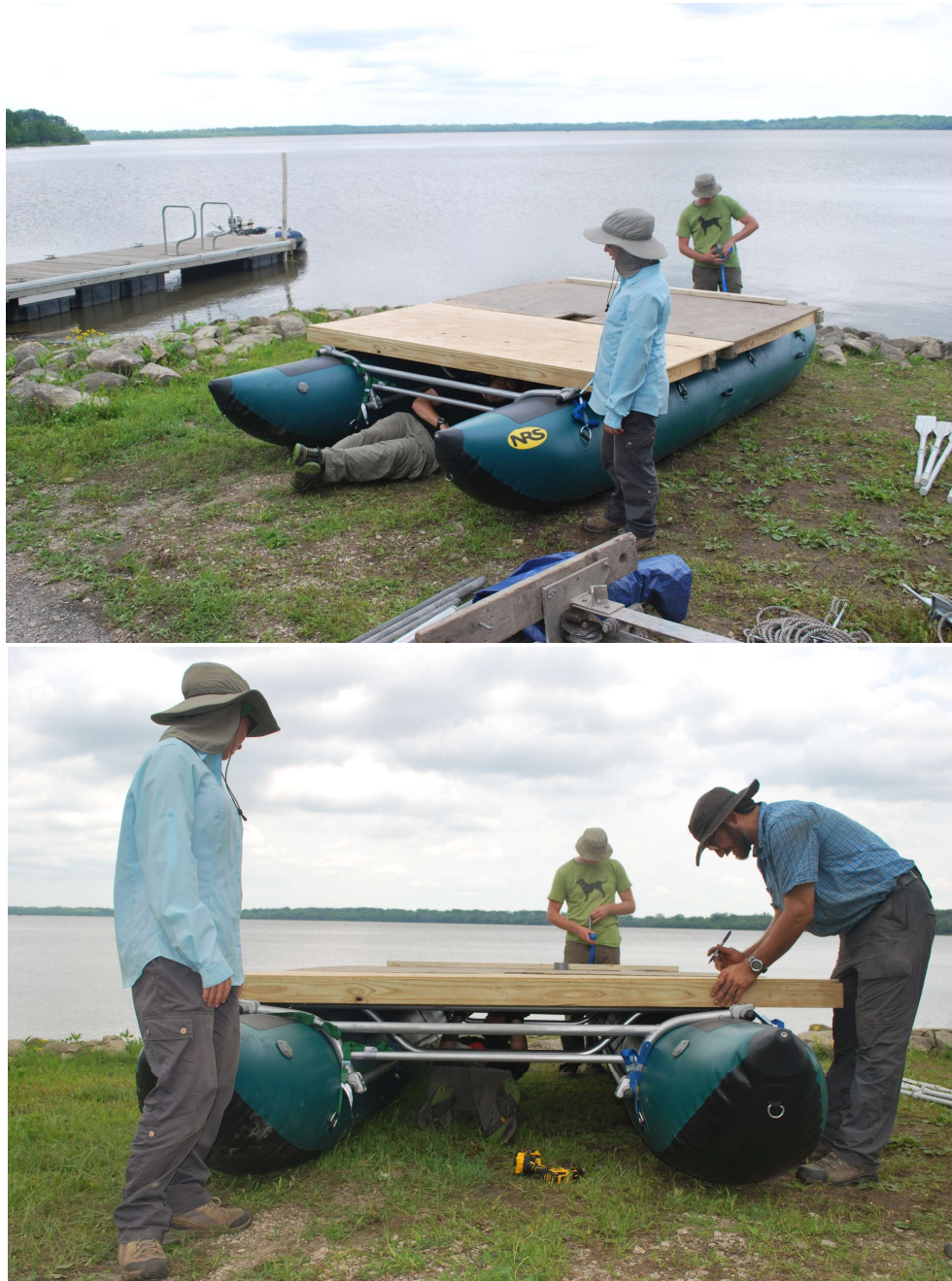
Figure 4.1 A wooden platform harnessed to inflatable tubes and aluminum Cataraft frame pictured here at Anderson Lake, Illinois, June 2014 (Photo by Caitlin Clark, 2014). This platform was also used at Hovey Lake, Indiana in July 2014.
