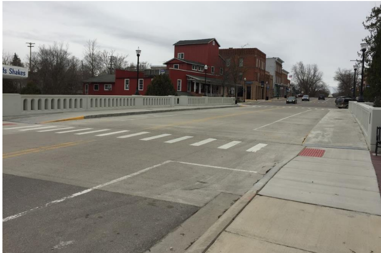
Figure 25: Manchester main street bridge with updated sidewalks. Photo Credit: Adam Jenks
