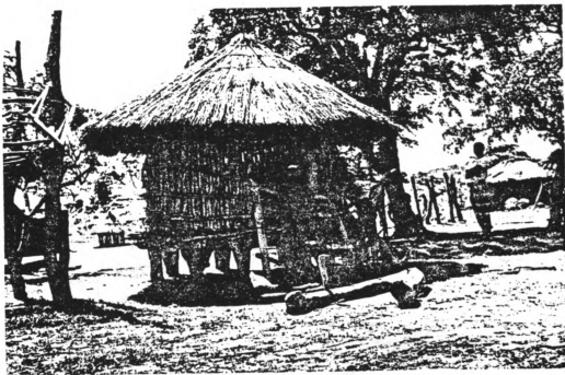
Figure 5.2 Timber Pole Type Maize (Cob) Store
