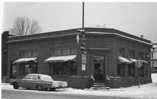
Figure 35.--First National Bank, Bayfield, 1905.
