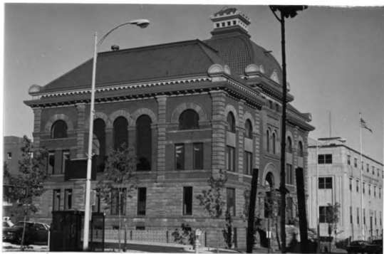
Figure 22.--Lovejoy & Demar, Marquette City Hall, Marquette, 1893-94.
