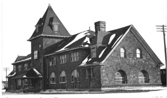
Figure 41.--Union Passenger Depot of the Wisconsin Central Railroad, Ashland, 1889.
