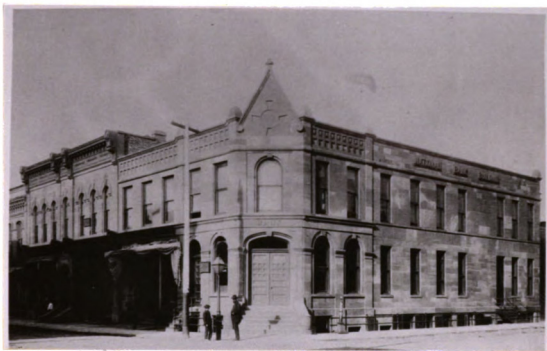
Figure 12.--Hampson Gregory, Superior Block, Marquette, 1885, destroyed.
