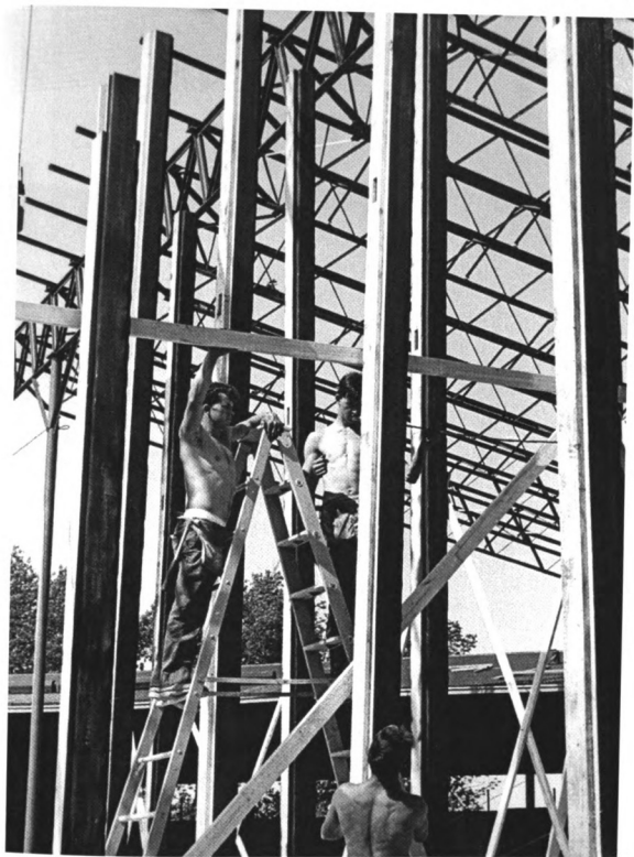
Figure 12 – Erection of Steel Beams in Stadium
