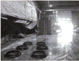
Figure 3.3. Steel Cage on the Bottom Ring
