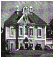
b. Residential Stucco Facade
