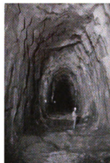
c. Tunnel Lining
