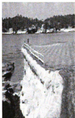
a. Shotcrete Retaining Walls
