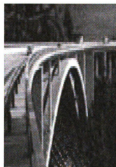
d. Bridge Decks
