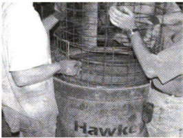
Figure 3.5. Adjustment of Steel Cage into Mold
