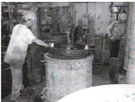
Figure 3.7. Placing the Tongue Mold Onto Concrete
