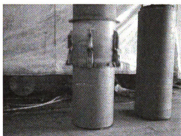
Figure 3.9. Immediate Demolding of Concrete Pipe
