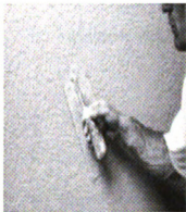
a. Application of Stucco
