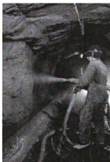
d. Structural Rehabilitation
