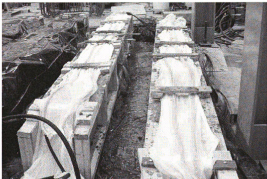
Figure 3.3 – View of HSC Beams after Fabrication
