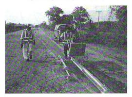
Figure A-3 Alligator Cracking on Site #6 (N5S-6)
