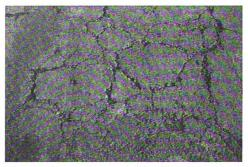
Figure 3.3 High severity fatigue cracking, N5S-6 (test site 6) (Wazirabad)
