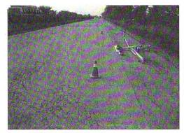
Figure A-2 Alligator Cracking on Site #5 (N5N-5)
