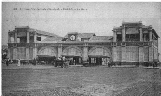
Figure 2.12 [The train station in Dakar, postcard located in the Annex of the ANS.]
