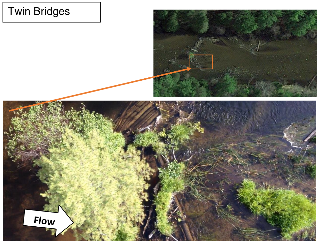
Figure 1.9: Close-aerial photo of Twin Bridges structure, top: satellite image with photo outline
