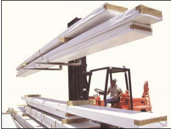
Figure 2.15: Unloading of Glulam Beams (Source: APA, 2013)
