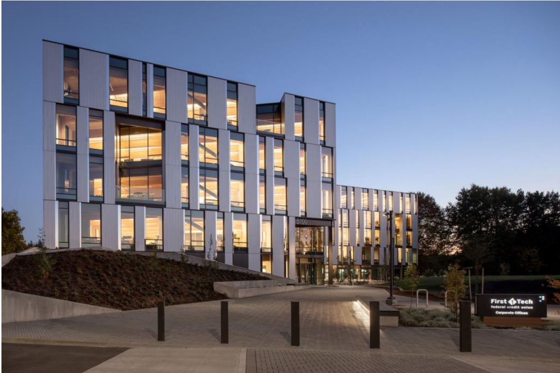
Figure 1.10: First Tech Federal Credit Union Project (Source: Swinerton Mass Timber)
