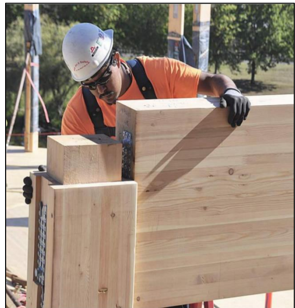
Figure 2.24: Prefabricated Post-to-Beam Connection (Source: MyTiCon Timber Connectors, 2019)
