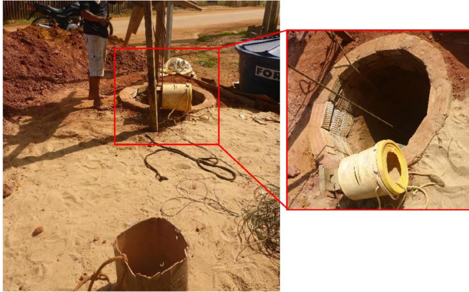
Figure 3.6: “Well digger” making a household well.
