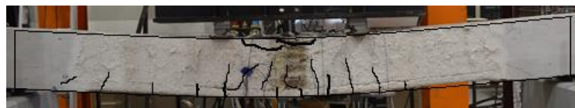
(f) Beam B2 at failure
