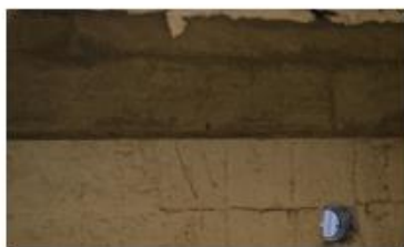
Typical beam just prior to fire exposure
