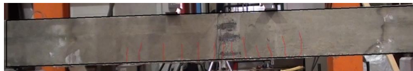
(d) Beam B4 at the beginning of residual tests
