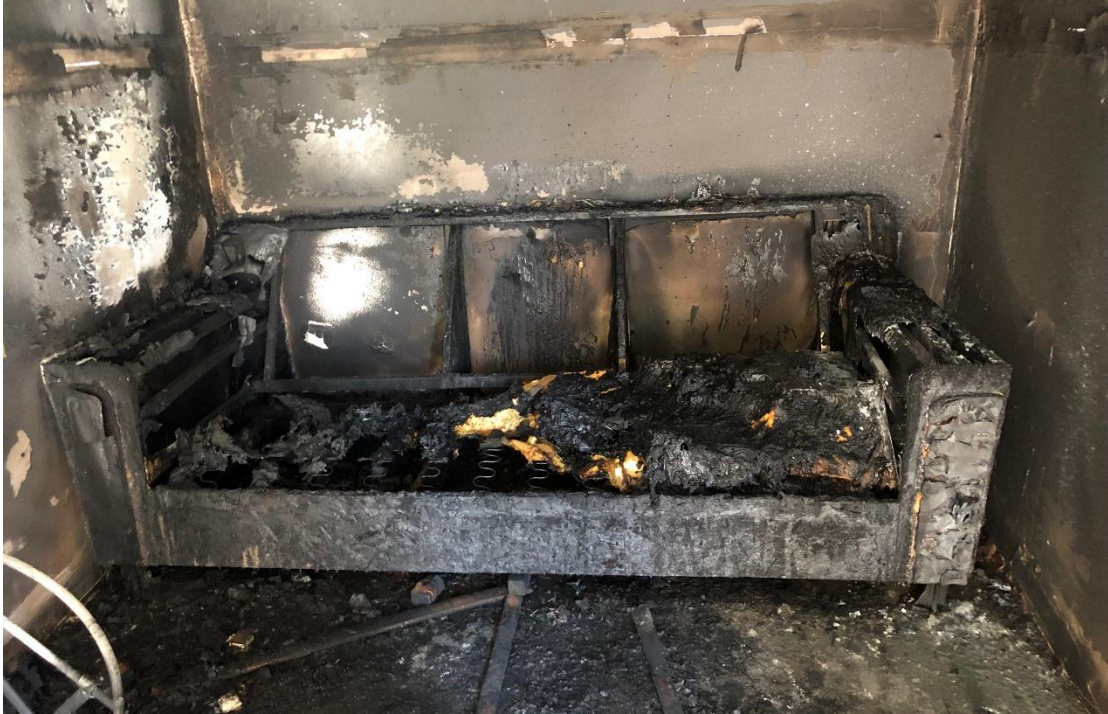
Figure A.3 Burned couch and debris inside burn cell post-burn
