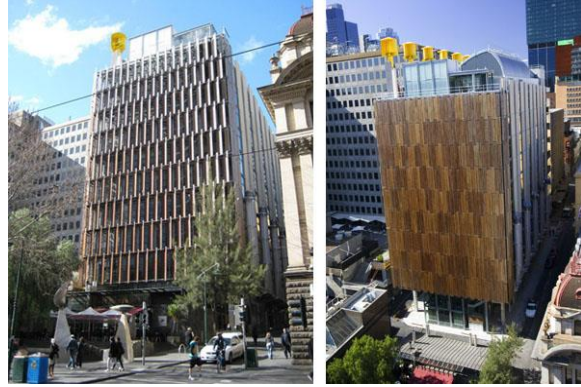
Figure 2-2. The façade is opened (left), and the façade is closed (right). From “Council House 2,” by City of Melbourne, 2010.
