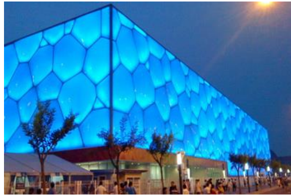
Figure 2-4. The assembly stem of the vertical surface made from ETFE. From “China.org.cn,” on Beijing 2008, 2006.
