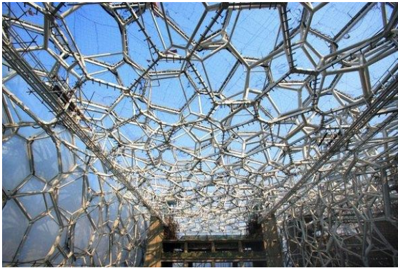
Figure 2-3. The Beijing National Aquatic Center has a design of bubbles enclosing the building that is based on the Weaire-Phelan structure. From “China.org.cn,” on Beijing 2008, 2006.
