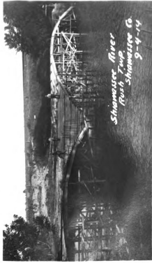
SIDE ELEVATION OF FORMS
