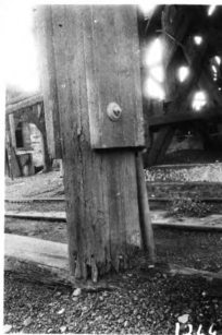
Figure 4.- Decay on coal tipple timbers at points of contact. (Courtesy The Barrett Company)
