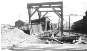
Figure 11.- Two creosoting tanks at an Indiana mine, West of Vandalia. Built of concrete and equipped with coils to give hot and cooling treatment. (Courtesy The Barrett Company)
