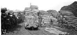
Figure 7.- A mine timber yard. Shows supply carried on hand and also shows men loading a mine car with timbers to be used in timbering operations in the mine entries. (Courtesy The Barrett Company)
