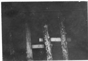
Figure 5.- Dry rot fungus fruiting bodies on cross bar timbers in main entry of mine 250 feet below ground. (Courtesy The Barrett Company)
