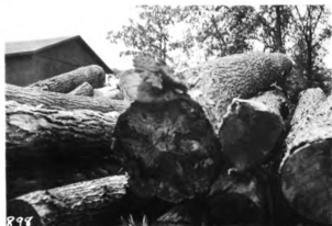
Figure 1.- Fungus fruiting bodies on cross bar timbers in timber storage yard. (Courtesy The Barrett Company)
