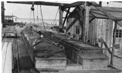
Figure 10.- Hot and cold treating tanks built of wood lined with metal. A good type for mines. (Courtesy The Barrett Company)
