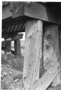
Figure 2.- Decay on surface mine structures above ground. (Courtesy The Barrett Company)
