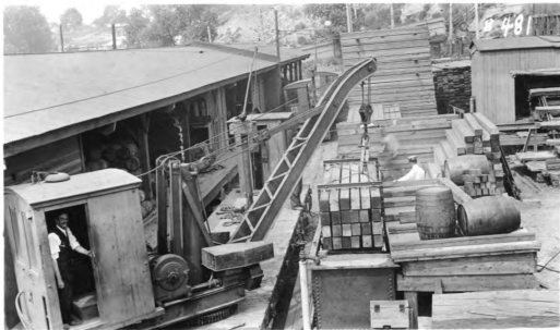
Figure 9.- Lowering rack of ties into the tank containing hot creosote. (Courtesy The Barrett Company)
