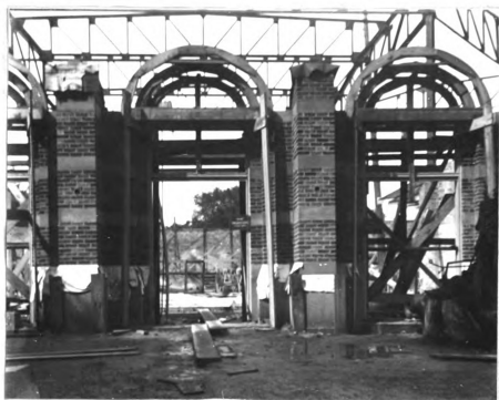
Entrance during construction, showing forms for door-ways, also the steel roof frames in the background.
