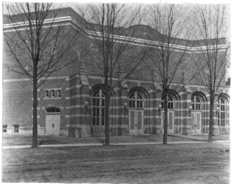
Entrance and portion of South-east side.
