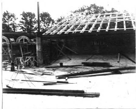
South Balcony during construction
