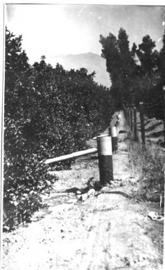
Stand pipes with leads of pipe extending down the rows.
