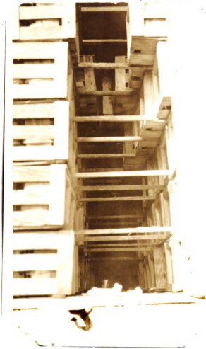
Poorly-Braced Car of Georgia Peaches
