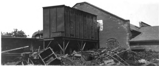
Fig. 12. Dust collector. There are several screens and a shaker motor in this housing. The air is drawn through and cleaned before going to the fan so no dust passes through the fan.
