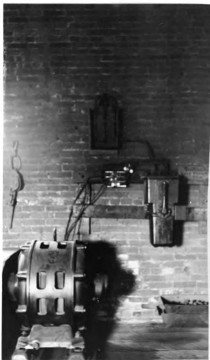
Fig. 17. Tumbler Motor and wiring. This is fed from the pole shown in Fig. 7. out in the court.
