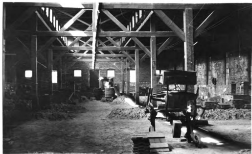
Fig. 15. North Foundry. This and the core rooms of similar construction were built within the last year or so.
