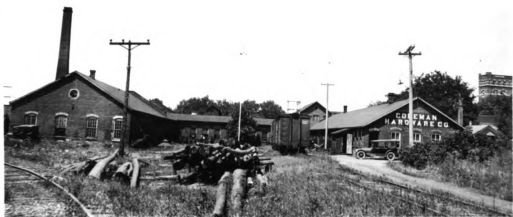
Fig. 1. General view looking west. Top of transformer rack can be seen over freight car. See blue print sketch 2.
