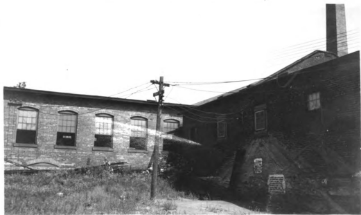
Fig. 7. Outside distribution center looking east toward Steel Room. Size of these wires should be increased and installed in a workman like manner using proper insulators, cross arms &c.
