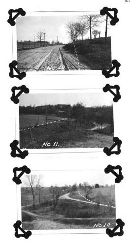
The 8% grade at sta.95 is reduced to 5% by making use of a mound of earth at the left of the road, shown in photograph Nc.13, which offers one of the best proportunities for chear excavation on the whole project. This mound obstructs the view on the curve which is another reason for its removal and use as a fill.
