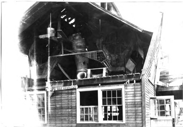
RESULT OF EXPLOSION IN ONE OF THE EARLY SULPHUR GRINDING EXPERIMENTS
