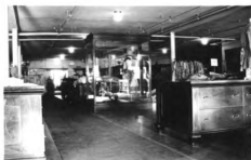
Second Floor - South Side
