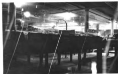
Basement - South Side.
