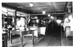
Second Floor - North Side
