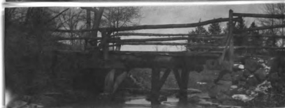
No. 215. w. pk. hw. br. 27' l. x 15' wd. abut. st. cn poor h. a. w. 4' str. 20' wd. x 2' d., f. banks sloping
