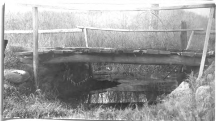
No. 184. w. pk. hw. br. 11.4' l. x 14.2' wd. abut. w. cn poor h. a. w. 3' str. 9' wd. x 5' d., f. banks low and sloping
