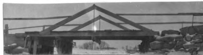
No. 35 \frac{1}{2} . w. k.p. hw. br. 22' l. x 14' wd. abut. st. cn good h. a. w. 6' str. 20'wd.x5'd.,n.f. banks low fill 2'h. x 1000' l.
