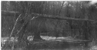
No. 117. w. pk. hw. br. 8' l. x 12' wd. abut. st. cn poor h. a. w. 2.9' str. 6' wd. x 2' d., f. banks low and sloping
