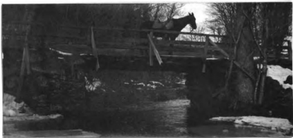
No. 101. w. pk. hw. br. 21' l. x 13' wd. abut. st. cn poor h. a. w. 7' str. 18' wd. x 2' d., f. banks sloping
