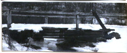
No. 152. w. pk. hw. br. 13' l. x 11' wd. abut. st. cn poor h. a. w. 3.6' str.8'wd.x1.6'd.,f. banks low
