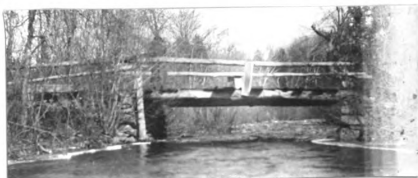
No. 33. w. pk. hw. br. 23.6' l. x 11.8' wd. abut. st. cn fair h. a. w. 4.2' str. 24'wd.x2.5'd., f. banks sloping
