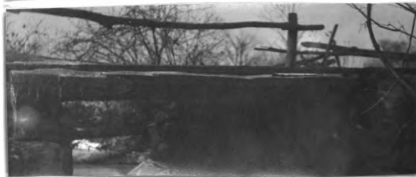
No. 199. w. pk. hw. br. 9' 1. x 14' wd. abut. st. cn poor h. a. w. 5' str. 6' wd. xl' d., f. banks sloping
