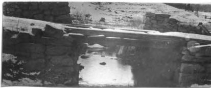
No. 77. w. pk. hw. br. 11.10' l. x 13.10' wd. abut. st. cn poor h. a. w. 3.8' str. 12' wd. x 1' d., f. banks low and sloping
