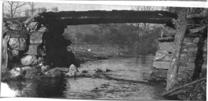
No. 188. w. pk. hw. br. 20.9' l. x 13' wd. abut. st. cn good h. a. w. 9.7' str. 15' wd. x 2' d., n. f. banks low and sloping
