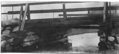
No. 7. w. pk. hw. br. 11' l. x 16' wd. abut. st. cn poor h. a. w. 4.9' str. 8' wd. x 3' d., n.f. banks low and marshy
