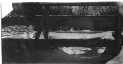
No. 105. w. pk. hw. br. 12' l. x 12' wd. abut. st. cn good h. a. w. 4' str.10'wd.x1'd.,f. banks sloping
