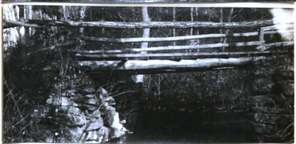
No. 151. w. pk. hw. br. 14.9' l. x 14' wd. abut. st. cn good h. a. w. 6.9' str.10'wd.x1'd.,f. banks sloping
