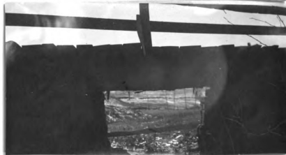
No. 226. w. pk. hw. br. 17.2' l. x 12.9' wd. abut. st. cn poor h. a. w. 6.7' str. 8' wd. xl' d., f. banks sloping
