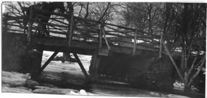
No. 62. w. pk. hw. br. 23.7' l. x 18' wd. abut. st. cn poor h. a. w. 8' str.20'wd.x1.6'd.,f. banks sloping
