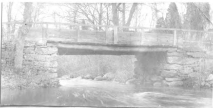
No. 12. w. pk. hw. br. 22' l. x 13.6' wd. abut. st. cn good h. a. w. 6.5' str. 20' wd. x 3' d., f. banks sloping
