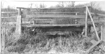
No. 186. w. pk. hw. br. 11' l. x 15.9' wd. abut. w. cn fair banks low
