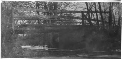
No. 213. w. pk. hw. br. 15.5' l. x 15.5' wd. abut. st. cn poor h. a. w. 7.8' str. 12' wd. x 2' d., f. banks low
