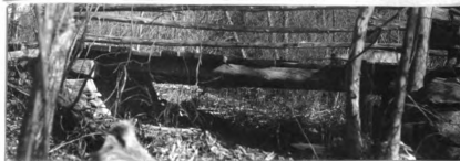
No. 128. w. pk. hw. br. 14' l. x 13.3' wd. abut. st. cn poor bottom dry banks sloping
