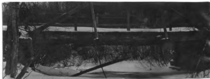
No. 8. w. q.p. hw. br. 33' l. x 13' wd. abut. st. cn good h. a. w. 7' str. 30' wd. x 3' d., f. banks sloping
