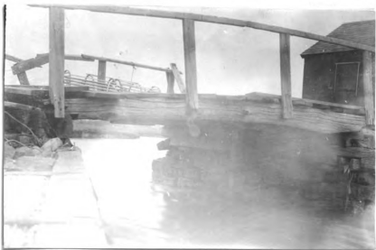
No. 61. w. pk. hw. br. 15' l. x 16.2' wd. abut. st. cn poor h. a. w. 5' str.12'wd.x5'd.,n.f. banks high and marshy
