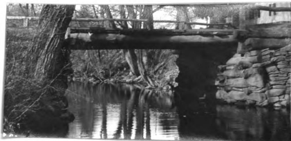
No. 182. w. pk. hw. br. 21.7' l. x 16' wd. abut. st. cn fair h. a. w. 6.5' str. 27' wd. x 1.8' d., f. banks low and sloping
