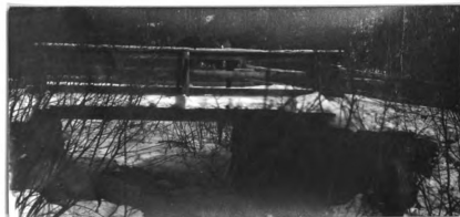
No. 157. w. pk. hw. br. 18.7' l. x 16.9' wd. abut. st. cn good h. a. w. 9.2' str. 15' wd. x 1.5' d., f. banks sloping
