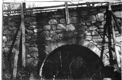
No. 176. st. Ar. hw. br. 20' l. x 18.3' wd. abut. st. cn good h. a. w. 20.7' str. 20' wd. x 1' d., f. banks low and sloping
