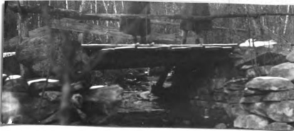
No. 133. w. pk. hw. br. 9'l. x 13.5' wd. abut. st. cn poor h. a. w. 4' str.11'wd.x1'd.,f. banks low
