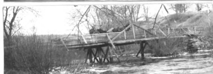
No. 34. w. k.p. hw. br. 70' l. x 14.6' wd. abut. st. cn good h. a. w. 7.9' str. 65'wd.x3'd.,n.f. banks sloping
