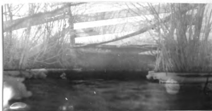
No. 111. w. pk. hw. br. 13.8' l. x 11' wd. abut. st. cn fair h. a. w. 2.6' str. 10' wd. x 1.8' d., f. banks low and marshy
