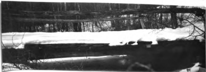
No. 156. w. pk. hw. br. 21' l. x 12.7' wd. abut. st. cn poor h. a. w. 2.5' str.15'wd.x2'd.,f. banks low
