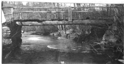
No. 174. w. pk. hw. br. 23' l. x 16' wd. abut. st. cn fair h. a. w. 6.8' str. 20' wd. x 2' d., f. banks sloping
