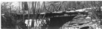
No. 126. w. pk. hw. br. 11.9' l. x 14.1' wd. abut. st. cn poor h. a. w. 3.9' str.10'wd.x1.6'd.,f. banks low
