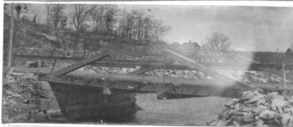
No. 89. w. q.p. hw. br. 46' l. x 11' wd. abut. st. cn good h. a. w. 8' str. 40' wd. x 4' d., n.f. banks sloping
