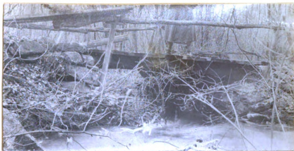
No. 149. w. pk. hw. br. 12.2' l. x 13.8' wd. abut. st. cn poor h. a. w. 3.5' str.10'wd.x2'd.,f. banks low
