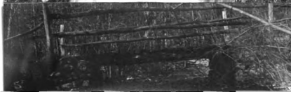
No. 130. w. pk. hw. br. 15.5' l. x 11.7' wd. abut. st. cn poor h. a. w. 4' str.10'wd.x2'd.,f. banks low
