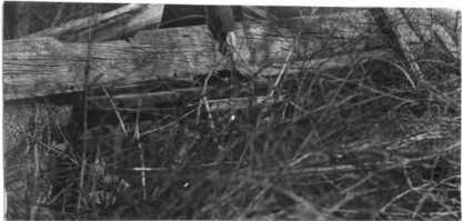
No. 44. w. pk. hw. br. 9.5' l. x 10' wd. abut. st. cn poor h. a. w. 3' str. 10' wd. x 1' d., f. banks low and sloping
