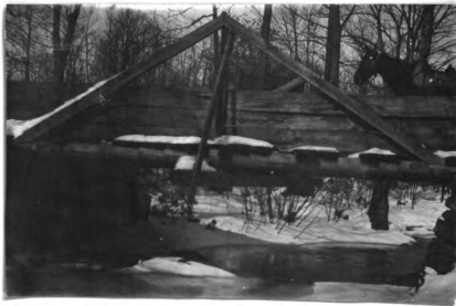
No. 97. W. k.p. hw. br. 23' l. x 13' wd. abut. st. on poor h. a. w. 7' str. 15' wd. x 1.6' d., f. banks sloping
