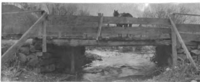
No. 104. w. pk. hw. br. 17' l. x 25' wd. abut. st. cn poor h. a. w. 4.6' str.16'wd.x1'd.,f. banks low
