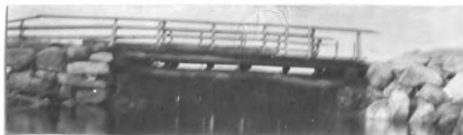
No. 6. w. pk. hw. br. 26' l. x 19' wd. abut. st. cn poor h. a. w. 5.8' str. 23' wd. x 4.6' d., n.f. banks low and marshy fill 3' h. x 550' l.
