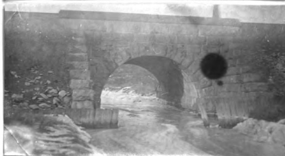
No. 30. st. Ar. R. R. br. 16.9' l. x 27.6' wd. abut. st. cn good h. a. w. 15' (arch) banks low fill 10' h. x 3500' l. height of track above arch 6'
