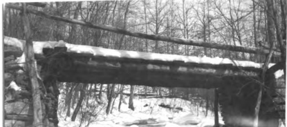
No. 128 \frac{1}{2} . w. pk. hw. br. 23' l. x 13' wd. abut. st. cn poor h. a. w. 9' str.8'wd.x2'd.,f. banks sloping
