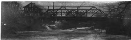
No. 75. s. Warren tr. hw. br. 34' l. x 15' wd. d. of gir. .5' abut. st. cn good h. a. w. 7.4' str. 25' wd. x 1.5' d., f. banks low
