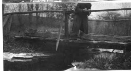
No. 35. w. pk. hw. br. 18.6' l. x 13.2' wd. abut. st. cn good h. a. w. 2.18' str. 10'wd.x1'd.,f. banks low and sloping
