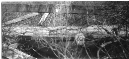
No. 43. w. pk. hw. br. 10' l. x 13' wd. abut. st. cn poor h. a. w. 2.1' str. 12' wd. x 1.8' d., f. banks low and marshy
