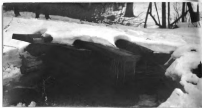
No. 193. w. pk. hw. br. 8.2' l. x 14.5' wd. abut. st. cn poor h. a. w. 6.2' str. 8.6' wd. x 1.5' d., f. banks sloping
