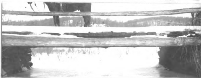
No. 131 \frac{1}{2} . w. pk. hw. br. 24' l. x 16' wd. abut. st. cn good h. a. w. 4.6' str.20'wd.x2'd.,n.f. banks low
