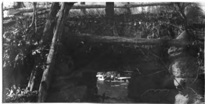
No. 40. st. hw. br. 12' l. x 10.5' wd. abut. st. cn good h. a. w. 3.5' str. 8' wd. x 2.5' d., f. banks sloping
