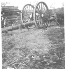
French Type of Big Wheels. Note narrow gauge and ponderous construction.
