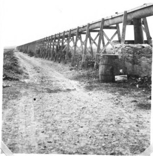
2. An irrigation flume.
