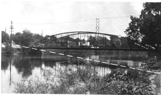
Old Boe String Truss to be Removed Dotted Line Showing Location of Proposed Structure.
