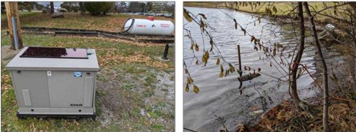
Figure 6.2: The propane generator (left) powers the aquarium heaters inside Gee's Minnow Traps (right).
