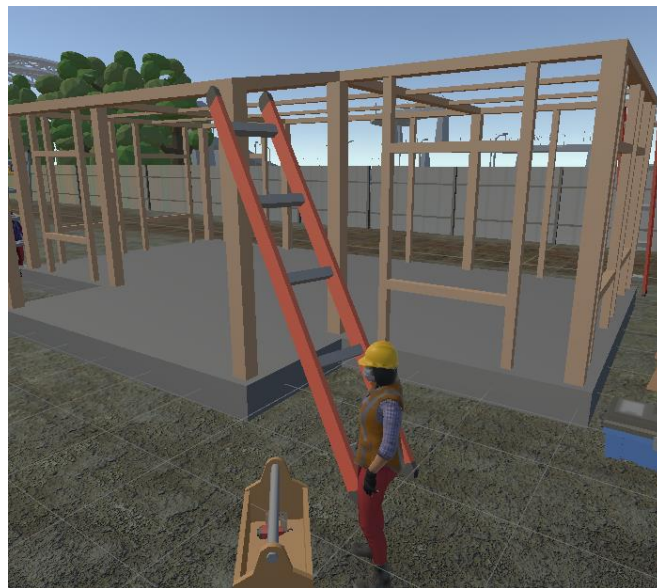
Figure 3.23: Hazard 4 – Base of ladder is too far from the edge of horizontal surface
