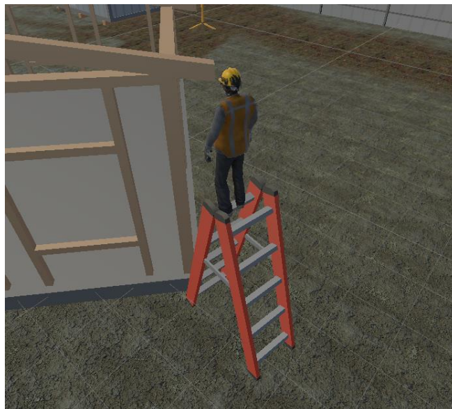
Figure 3.21: Hazard 2 – Worker standing on top rung of ladder
