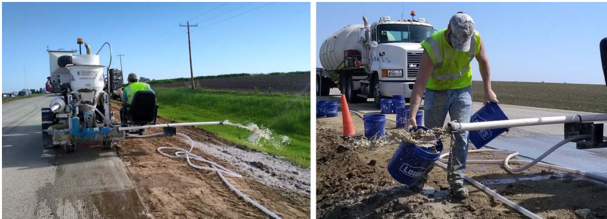
Figure 3: Direct Discharge CGR Collection (Site CGR-3 Shown), Photos by Patrick Bollinger
