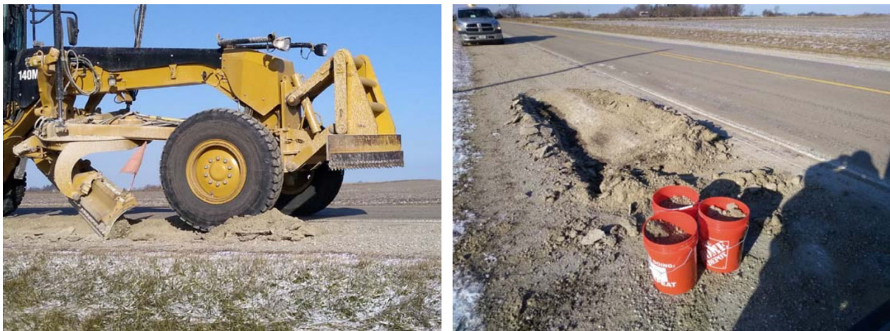
Figure 27: Motor Grader and Soil Sampling from CR G37 Located in Washington Co, IA, Photos by Patrick Bollinger
