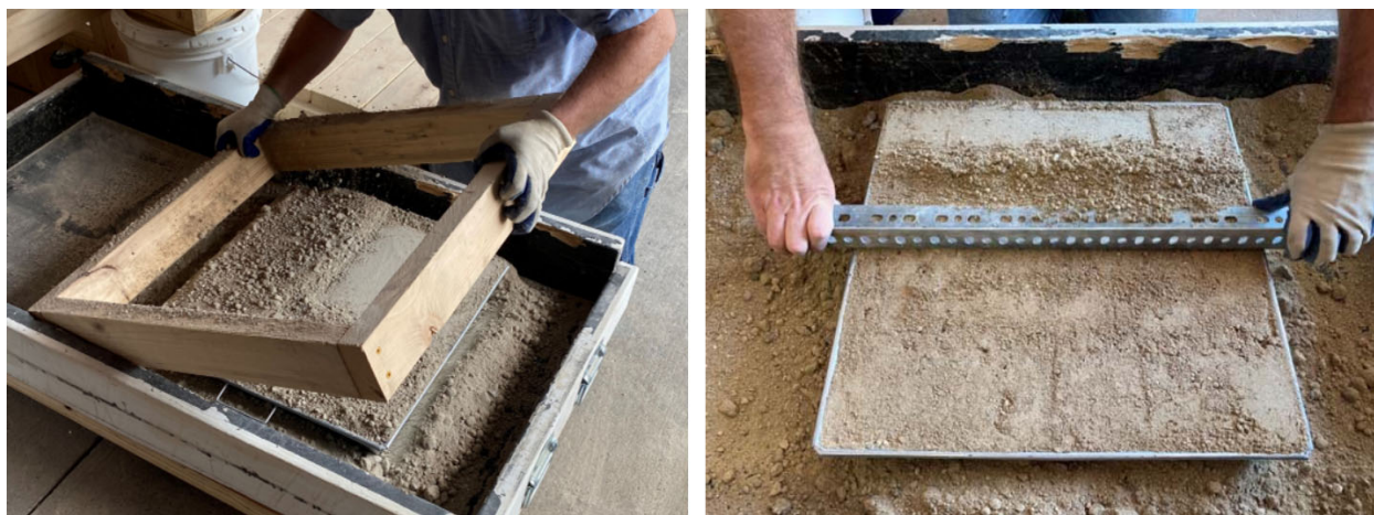
Figure 38: Preparation and Screeding of Compacted Soil Form, Photos by Patrick Bollinger
