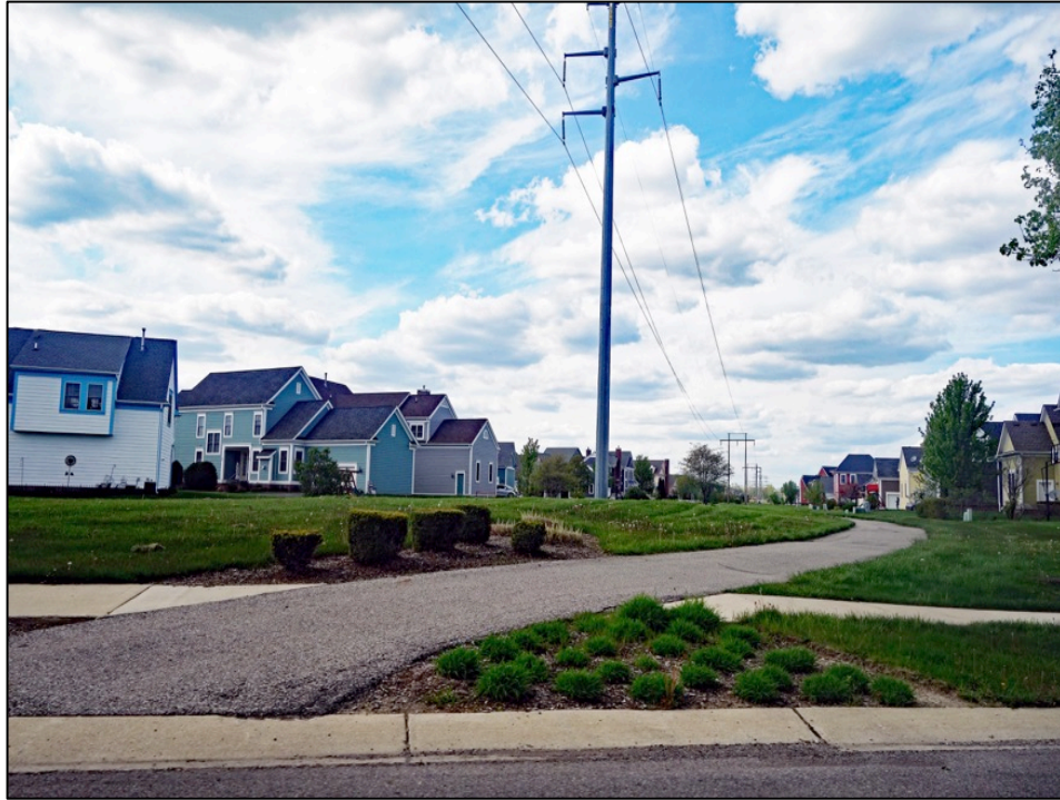
Figure 4.11: Power Lines Running through CHV Neighborhood (Image credit to author)
