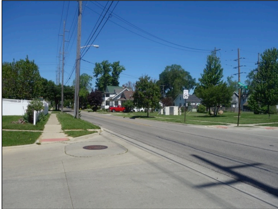
Figure 4.43: Absence of Safe Crossings for Pedestrians along Noble Street (Image credit to author)
