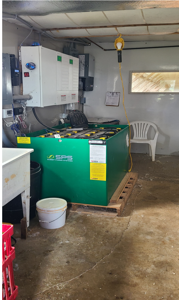
Figure 3.4: An array of batteries to power lights, fans and other technology at a barn.
