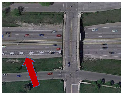
b. Chevron Markings at Ramp
