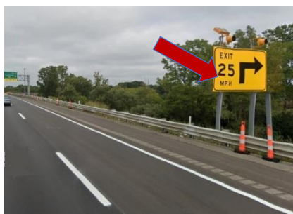
a. Flashing Ramp Warning Sign
