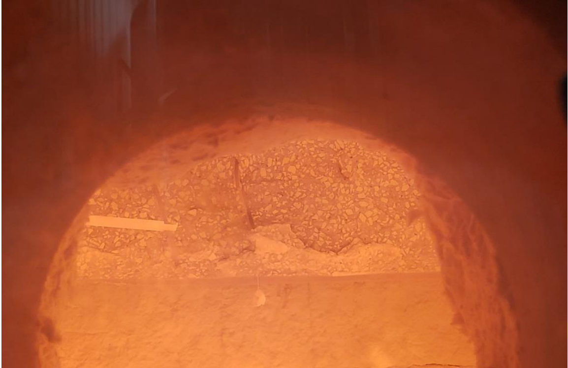
Figure C.5 Cracking and crushing of concrete in beam H1 at 40 minutes of fire exposure
