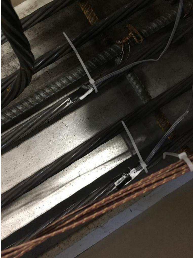
Figure C.2 Installation of strain gauges in PC beams at key locations
