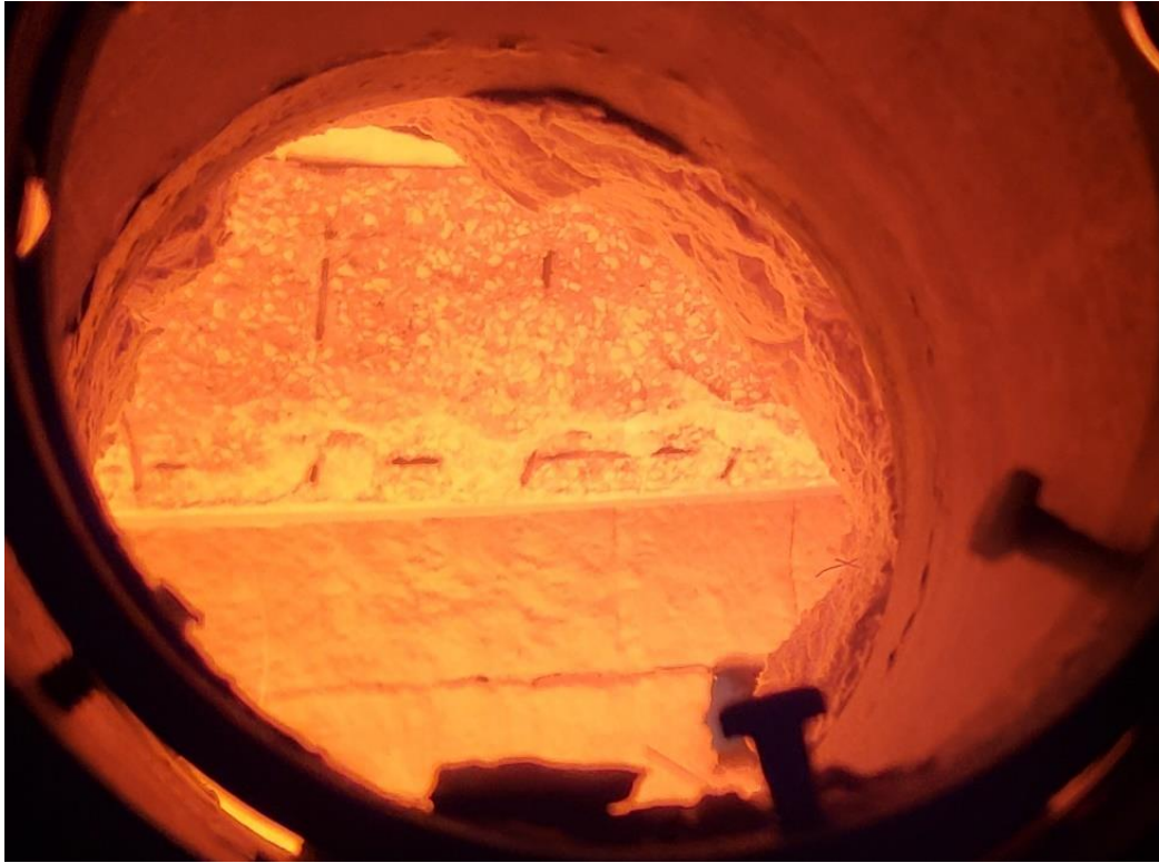
Figure C.6 Cracking and crushing of concrete in beam H1R at 40 minutes of fire exposure
