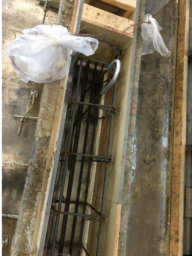
Figure C.1 Installation of thermocouples in PC beams at key locations
