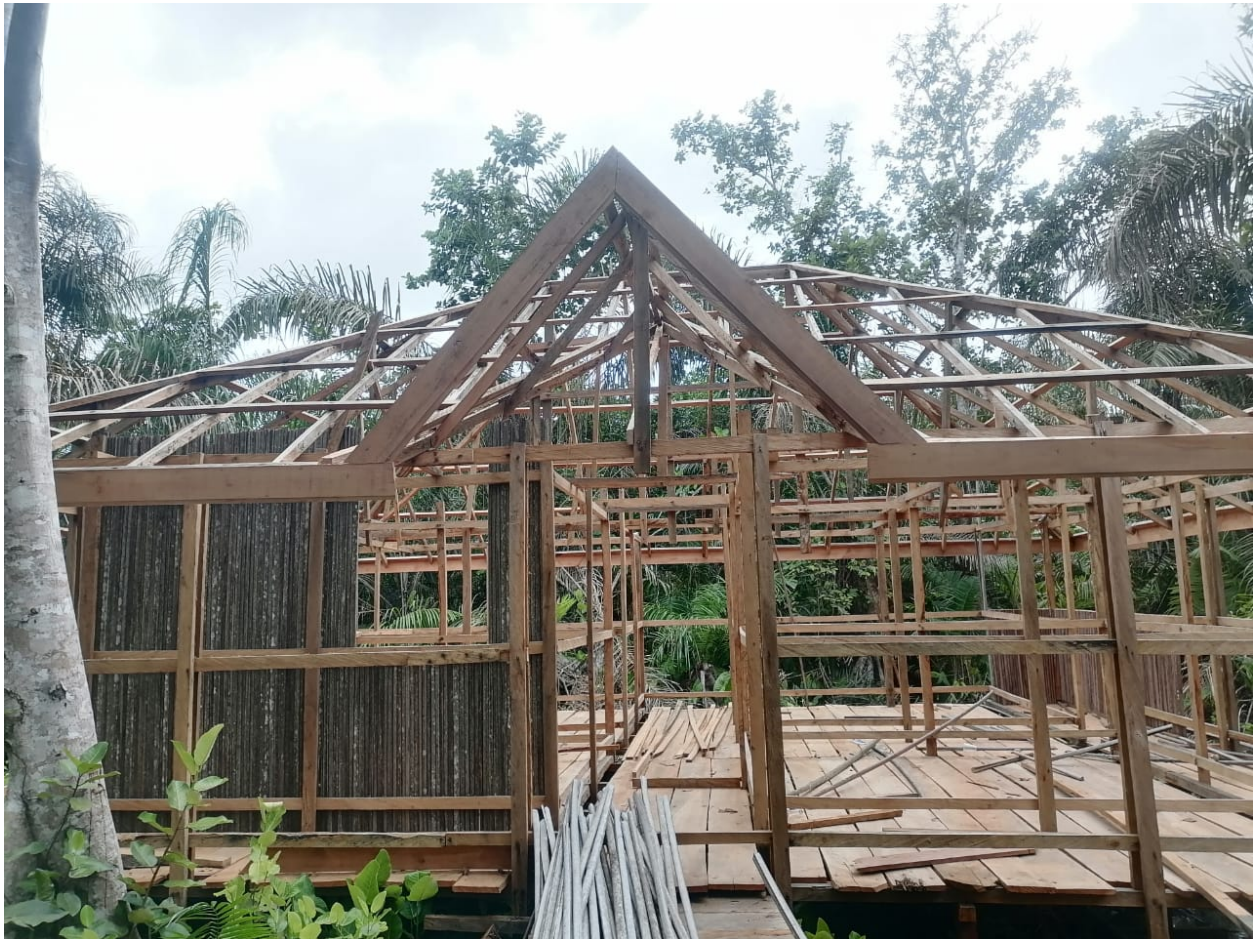
Figure 15: A Nzulezo House Structure Showing the Floorboard and Scaffold
