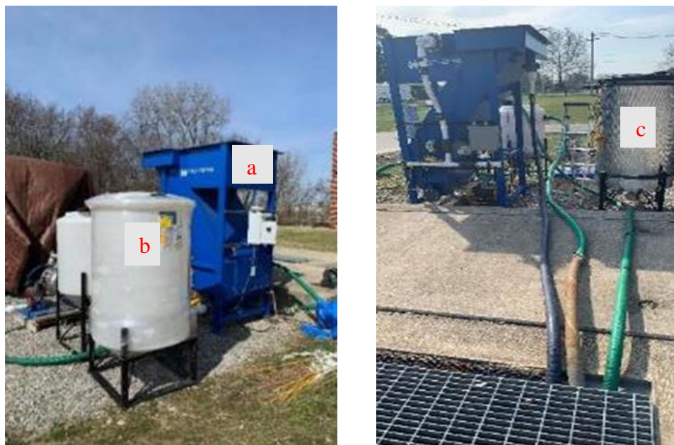
Figure 26. The blackwater setup. (a). The incline plate clarifier; (b). The sludge buffer tank; (c).
