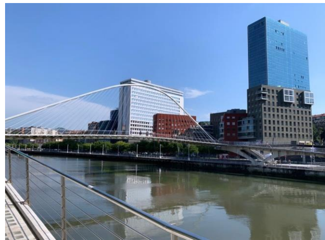
Figure 31: Zubizuri Footbridge Over the Nervión (Source: Nikolovski)
