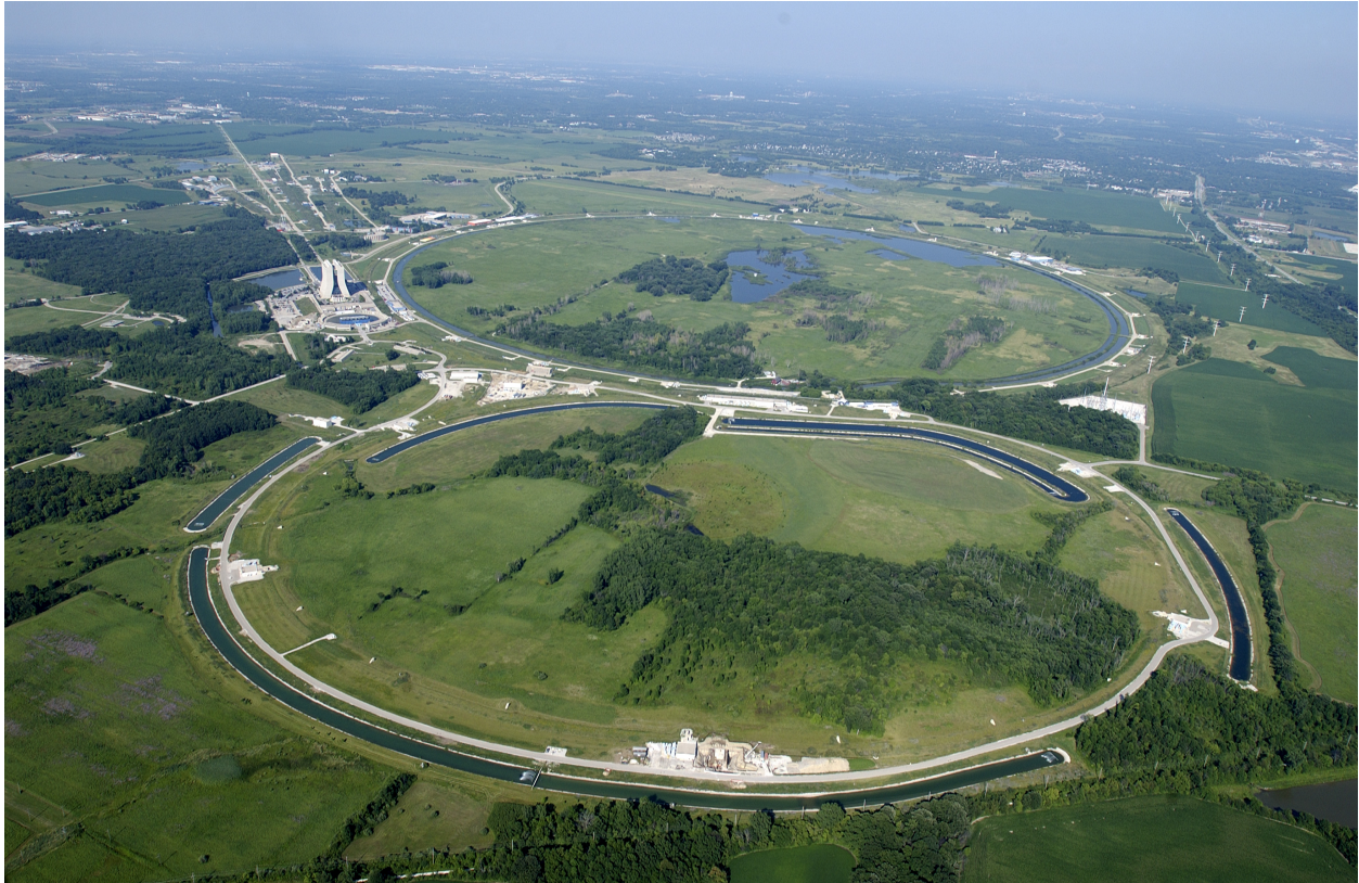
Figure 1.1 Aerial view of the Fermi National Accelerator Laboratory (FNAL) located in Batavia, IL, USA [11].
