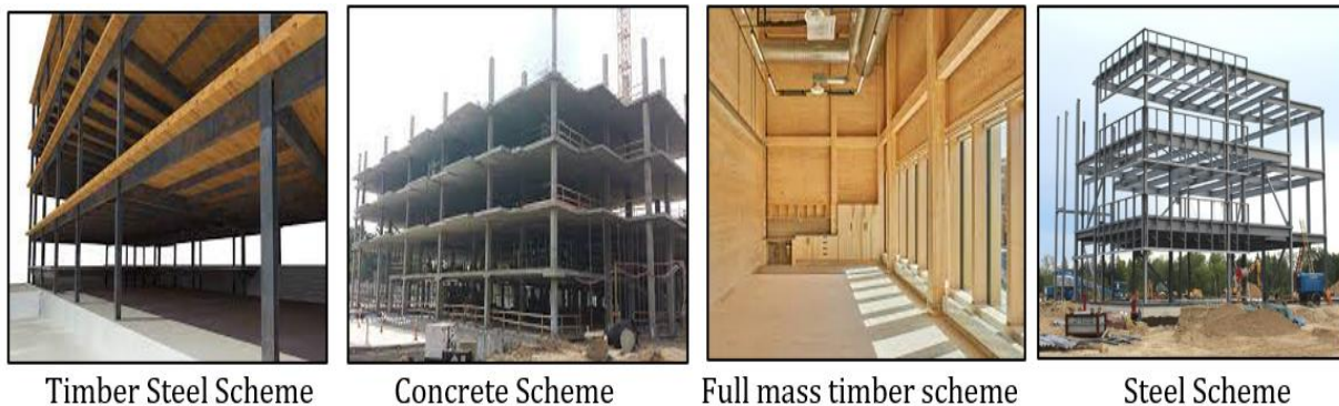
Figure 3.2: Different construction schemes for the case study
