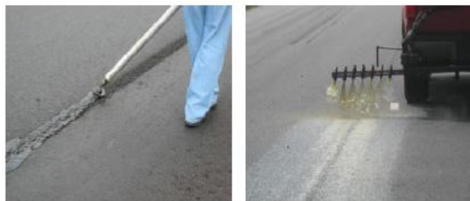
(e) Application of joint adhesive and sealants (14)
