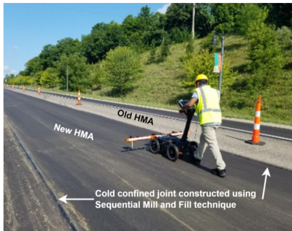
(a) Confined butt joints at M-45, MI
