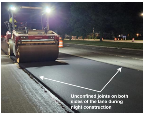
(a) Unconfined joints at M-102, MI
