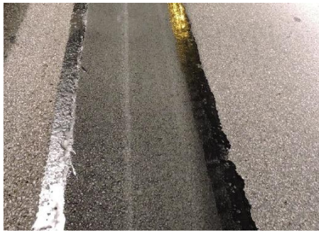
(a) Slot paving
