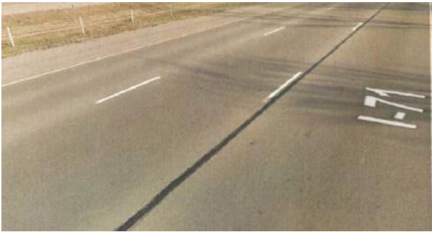
(c) Crack sealing
