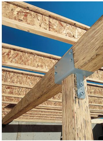
Figure 6 PSL beams (Woodworks 2021)
