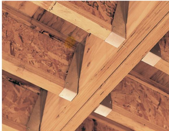
Figure 4 LVL beams (Woodworks 2021)
